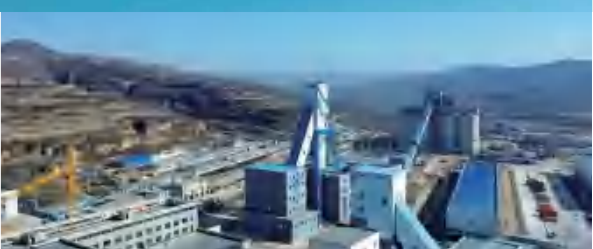
甘肃五举煤矿副立井
