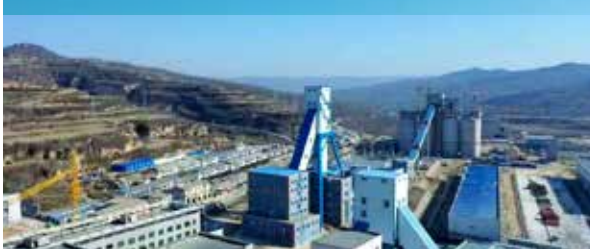
甘肃五举煤矿副立井
